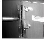
Install the fasteners with washers. For hinged door, position hinge on duct wall and plug weld.
