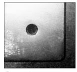
4b. CENTERED If you can not see the wall of the duct through any of the corner holes. then it is centered.
