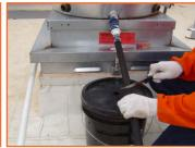
8. Measure and cut the hose allowing 2-3 inches extra for inside of the pail.
