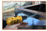
2. Install the Deflector Shield approximately 1/4" above the line drawn in step 1.
