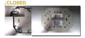
4. Once in place, turn fasteners clockwise to compress Access Armor Door to duct, creating an airtight seal. This completes your installation.
